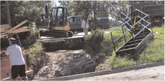
(Above) John Rupnicki (bottom left) and Anthony Levier (top) preparing the foundation for a new stairway that can be seen on the right. The stairway will allow pedestrians to go from the upper parking lot to the lower level parking lot on the west side of the Government Center.
