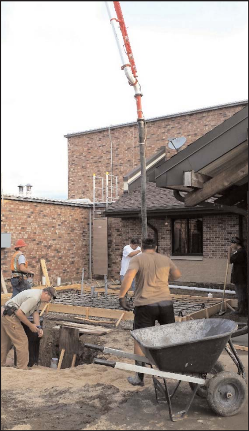
(Left to right) is Jim Harvey, an unidentified worker (in hard hat), Tom Jim, Gilbert Kent, and John Rupnicki preparing the foundation for the generator. Harvey, electrician for the PBPB, was connecting the anode bags for the underground propane tank.
