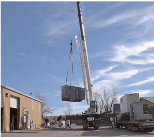
It took a semi truck to bring the generator to Road & Bridge and another crane truck to help install it on its base outside of the building. Later on, conduits were placed in the ground by the PBPN electrical team as one of the steps in getting the generator ready when it is needed in the future.
