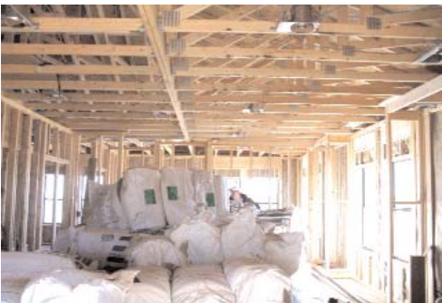
When this photo was taken Reservation Drywall was installing insulation in the pro shop inside the clubhouse.
