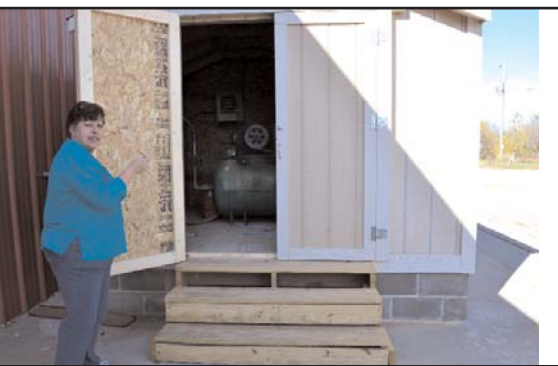
Brenda Pahmahmie, Road & Bridge Specialist, points to where a large air compressor has been placed in a shed outside the main building. Originally the compressor was housed in the kitchen of the main building that caused a lot of noise when it was used.
